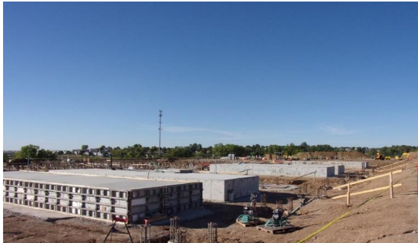
Facing Northwest – Engine Foundations
