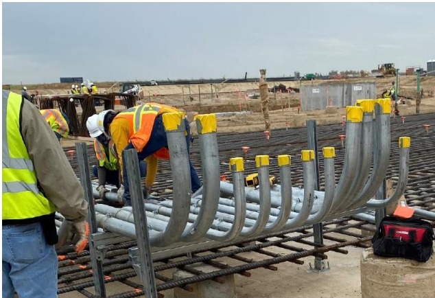
Facing East – Unit 2 Combustion Turbine Embedded Conduit
