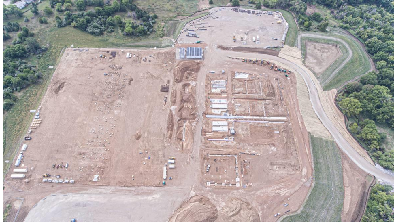
Facing South - Aerial view of site on 9/18/2022
