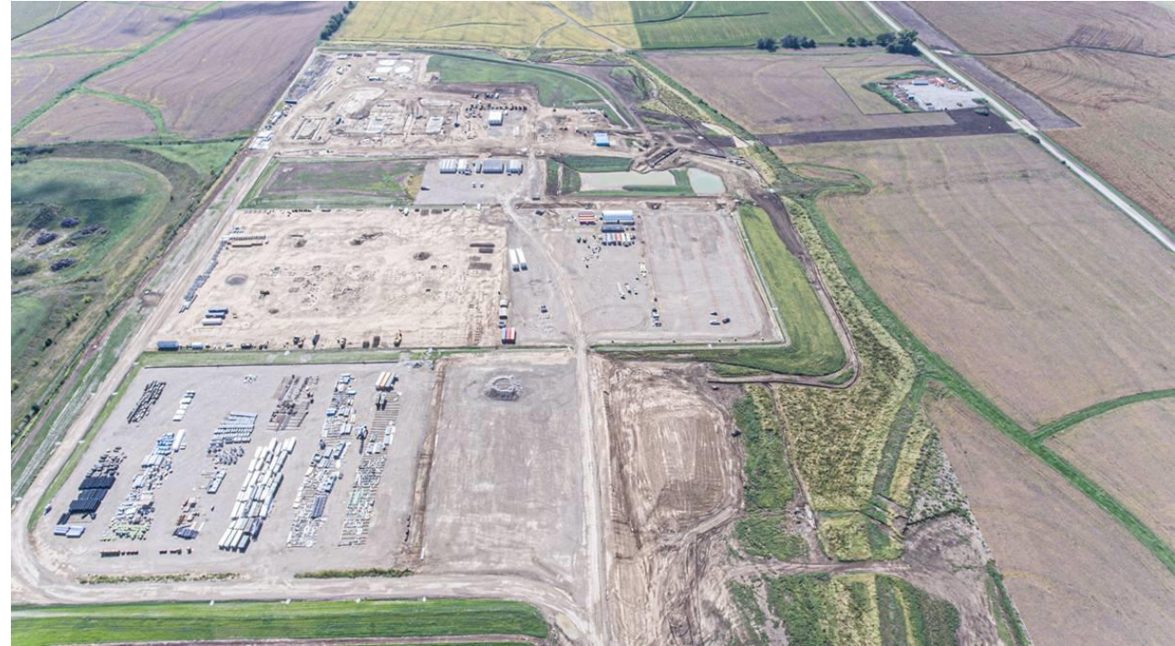
Facing South – Aerial view of site on 9/18/2022
