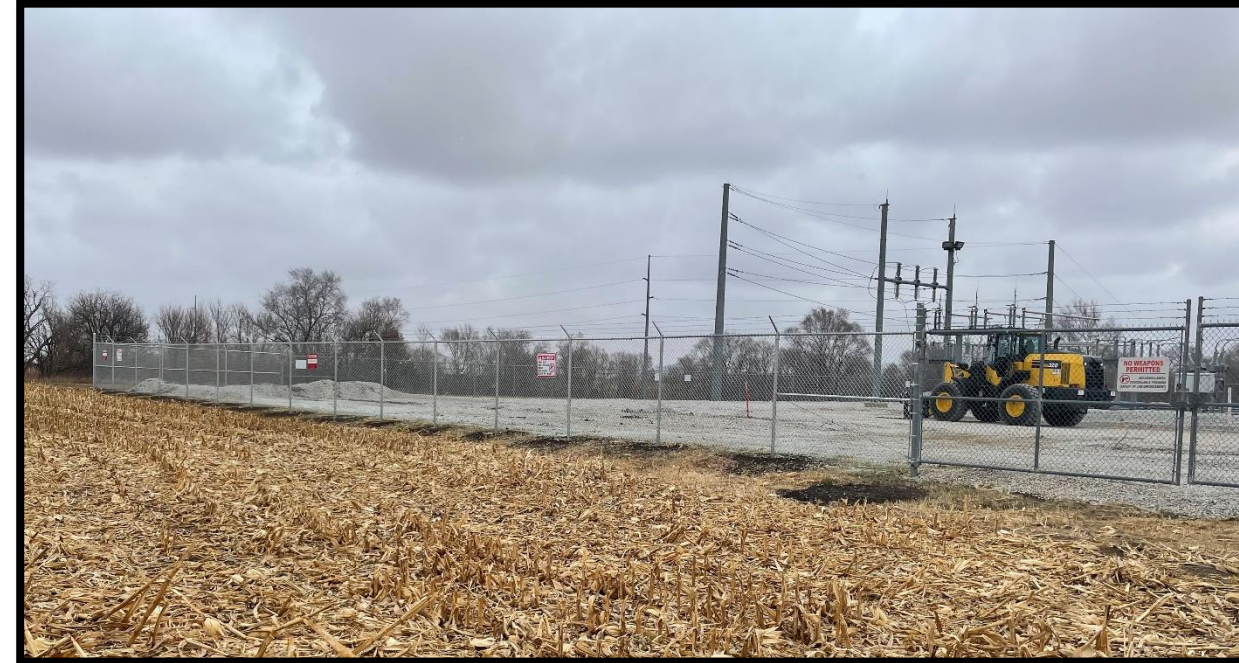
Construction work for interconnection at OPPD's substation
