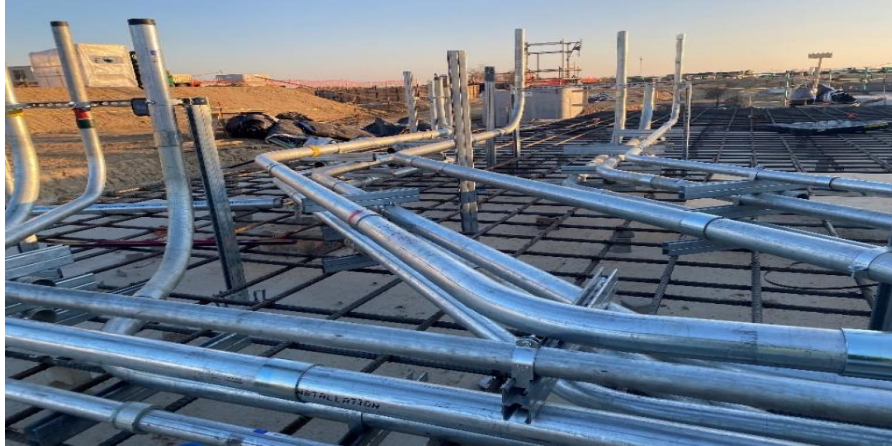
Facing SE - Unit 2 Gas Turbine Foundation Prep
