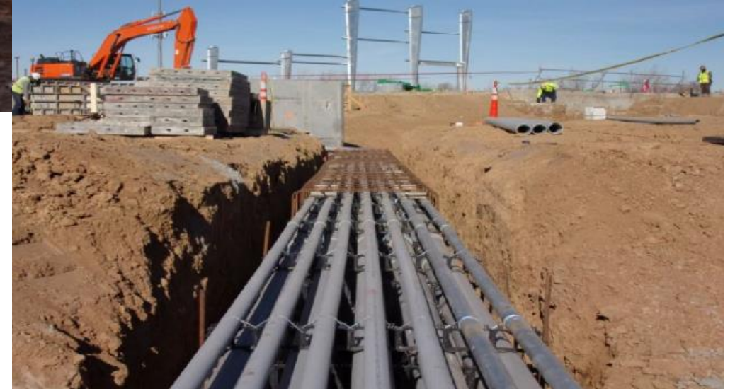
Duct Bank and Rebar for Road Crossing
