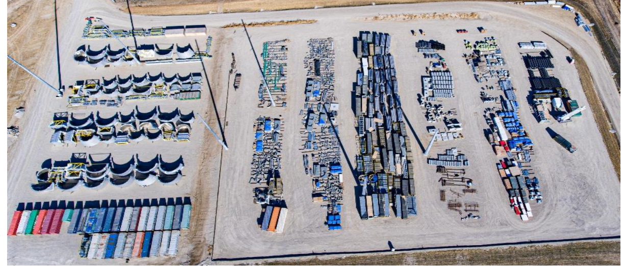
Facing North – Volume of Materials
