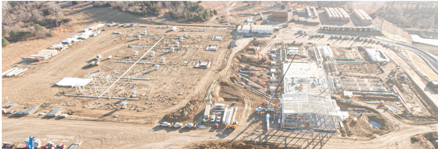
Facing South – Substation and Generation Construction Progress, 12/11/2022
