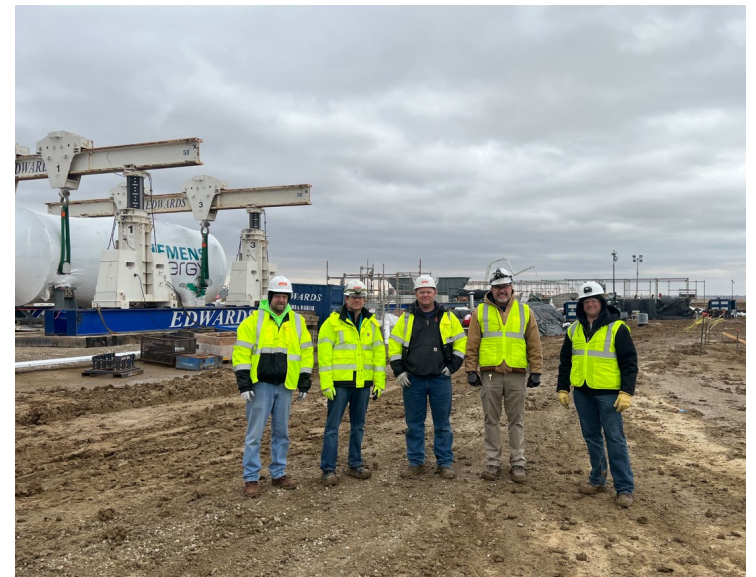
Gas Turbine #1, OPPD Staff Observance
