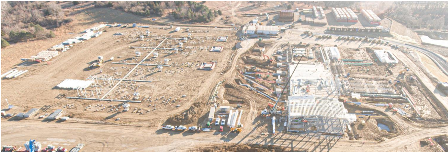
Facing South – Substation and Generation Construction Progress, 12/11/2022
