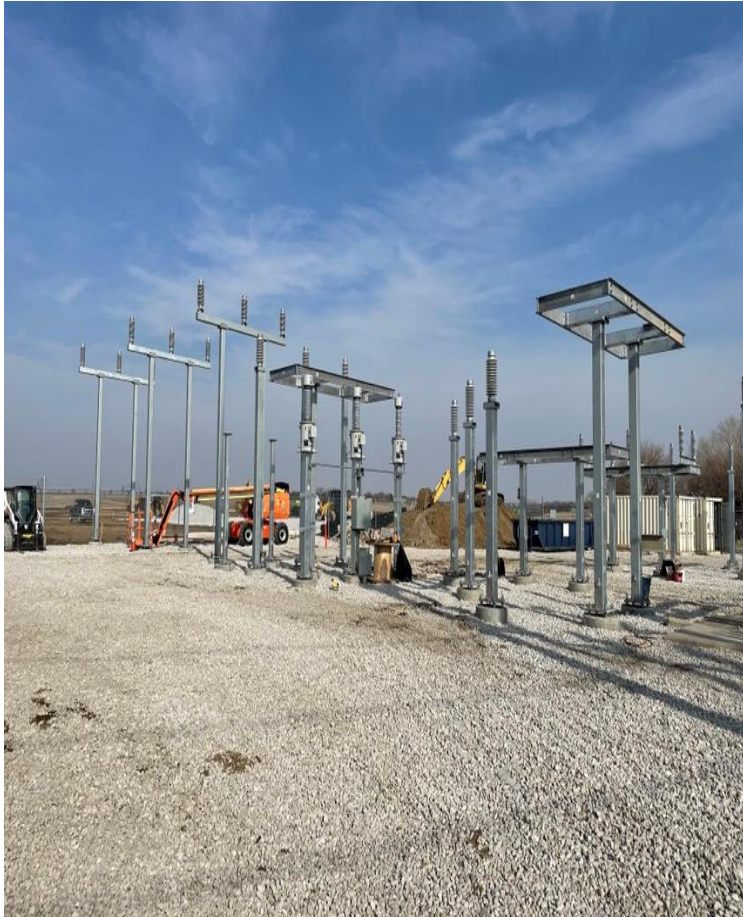
Substation – Construction Activities
