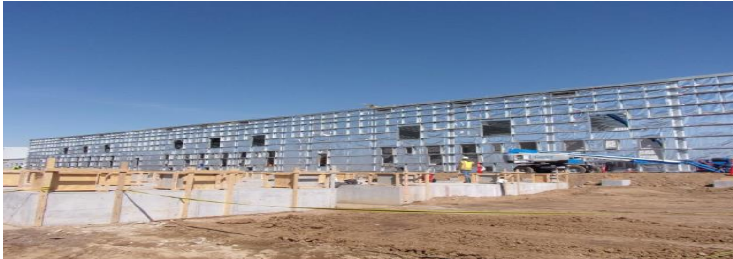
Facing Northeast – Engine Hall Enclosure
