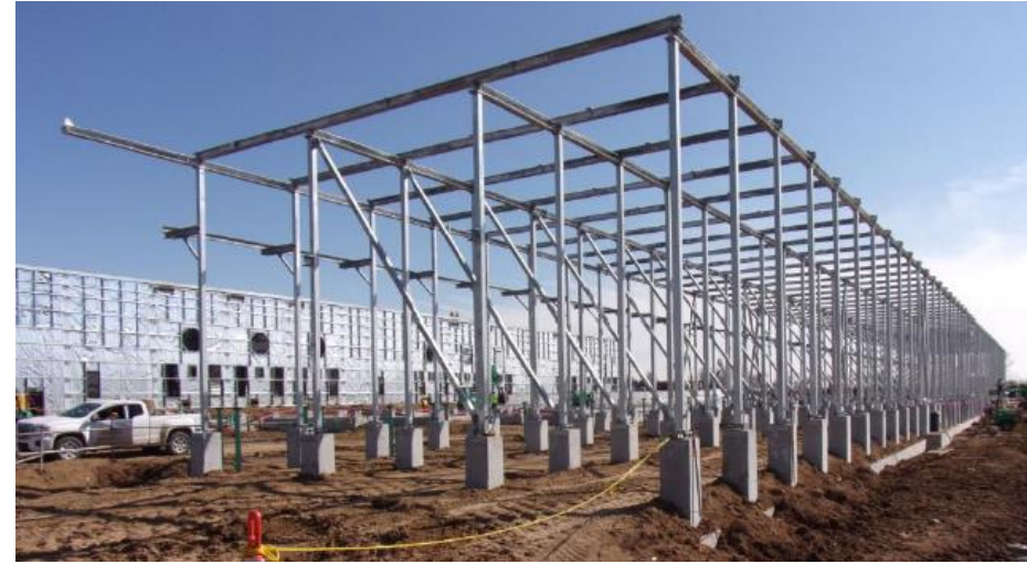
Facing Southeast – Radiator Structure
