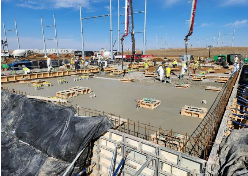
Facing Northwest – Power Distribution Center Foundation
