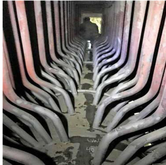
Reheater Outlet Header Inspection
