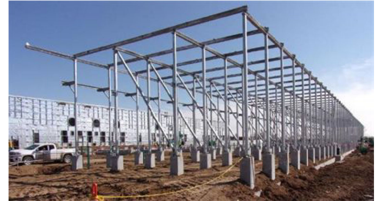
Facing Southeast – Radiator Structure
