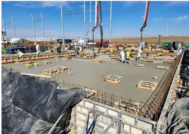
Facing Northwest – Power Distribution Center Foundation
