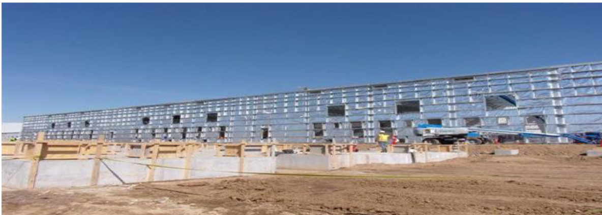
Facing Northeast – Engine Hall Enclosure
