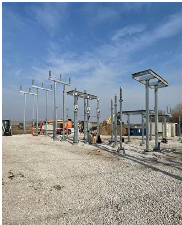
Substation – Construction Activities
