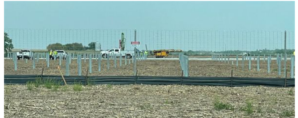
Platteview Solar – Piling Stands
