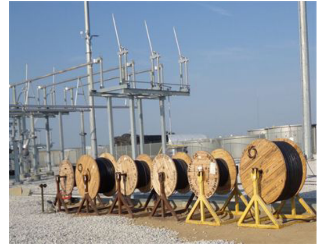
Substation - Cable Prep
