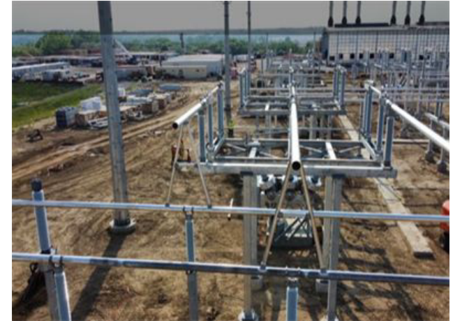
Facing West – Substation: Bus Installation
