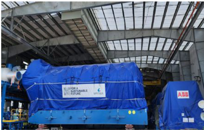
Facing North – Engine Hall
