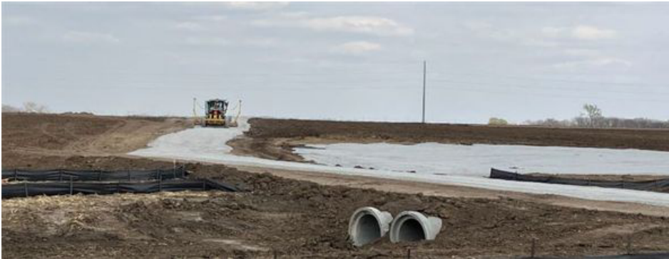
Platteview Solar – Access Road Preparations
