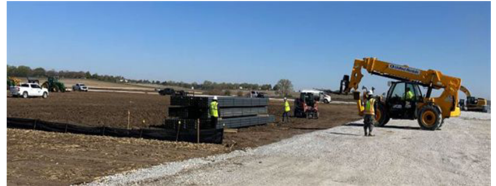
Platteview Solar – Material Staging
