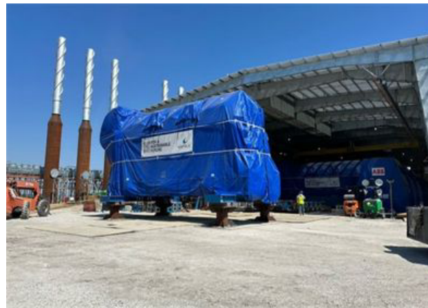
Facing Northwest – Engine Move to Hall
