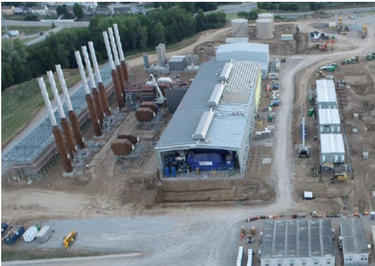
SBLs: Facing North, Aerial View
