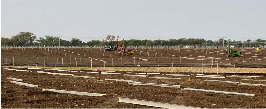
Platteview Solar – Pile Driving
