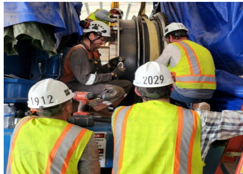
Engine/Generator Alignment/Coupling
