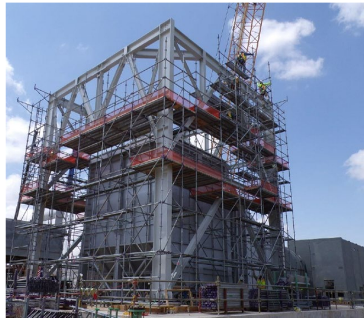
Facing Northwest – Unit #1 Stack Erection
