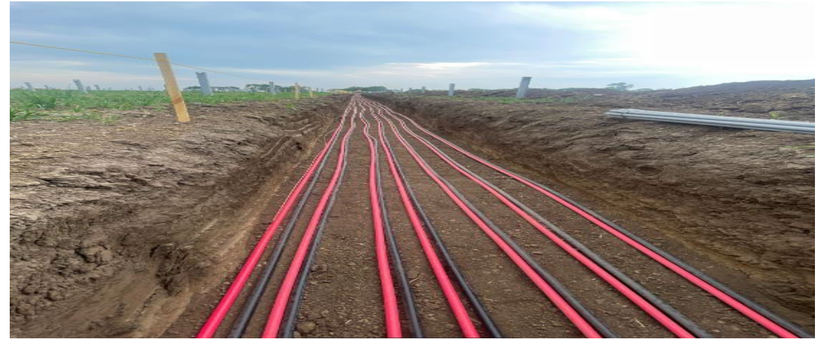
Platteview Solar – DC Trenching
