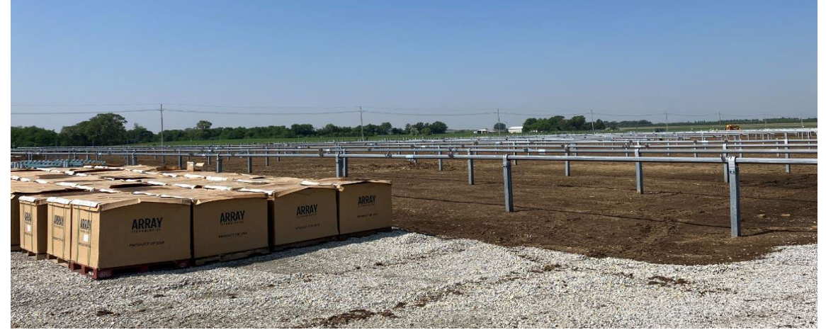
Platteview Solar – Racking Installation
