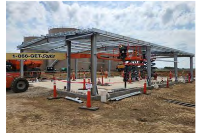
Fuel Building Erection
