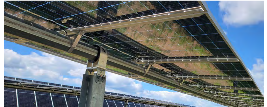
Platteview Solar – Racking & Module Installation
