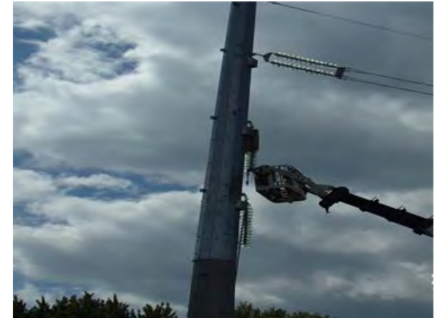
Substation Static Cable Mast Install
