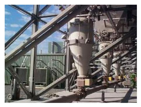
Example of new ash feeders and pneumatic transfer pipe
