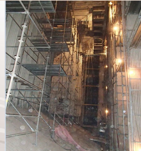
NC1 furnace slope replacement project
