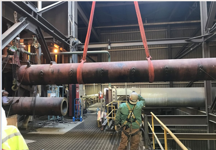
NC1 main steam header replacement
