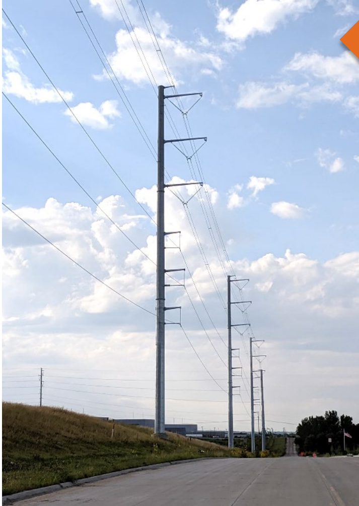
Double Circuit 345 kV/161 kV Monopole - Average height 165 feet - 6.7 miles
