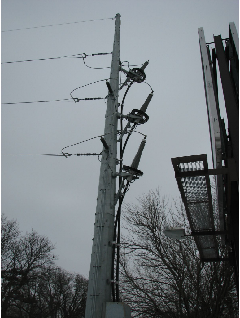
Transmission Cable Terminal Structure (EXAMPLE)
