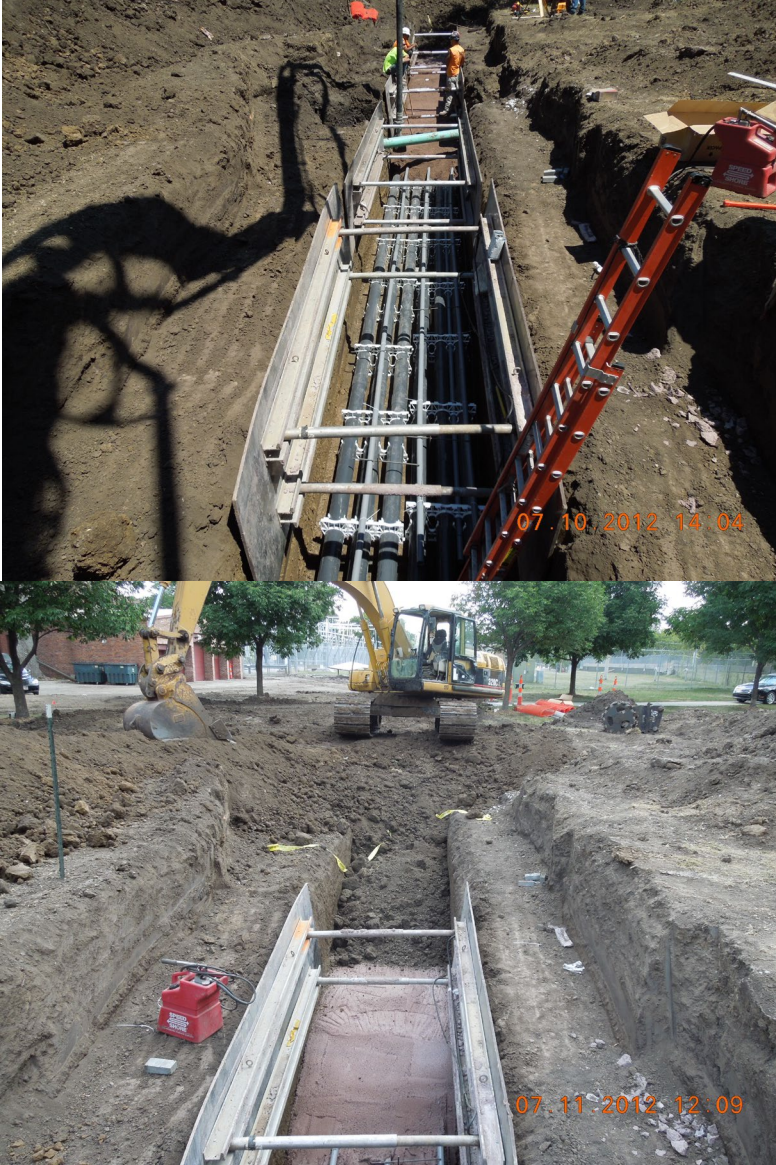
Ductbank Construction (EXAMPLE)
