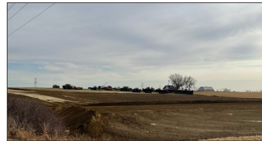
The substation is expected to begin operating in mid-2024.
