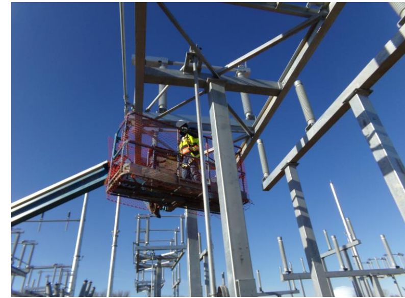
Substation – Horizontal Bus Installation
