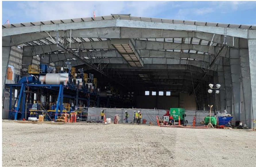
Facing North – Engine Hall Preparations & Installations
