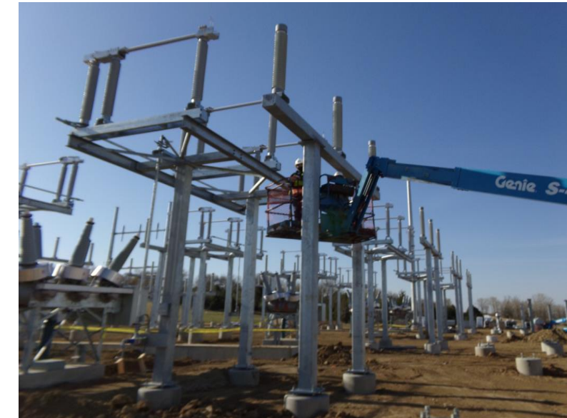
Substation – Horizontal Bus Installation
