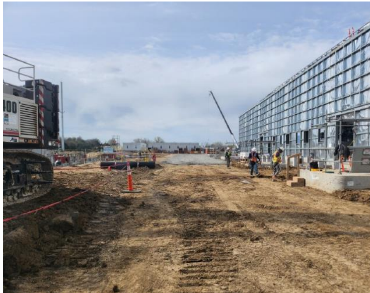
Facing South – On Site Heavy Haul Prep
