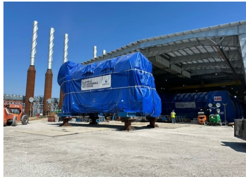
Facing Northwest – Engine Move to Hall
