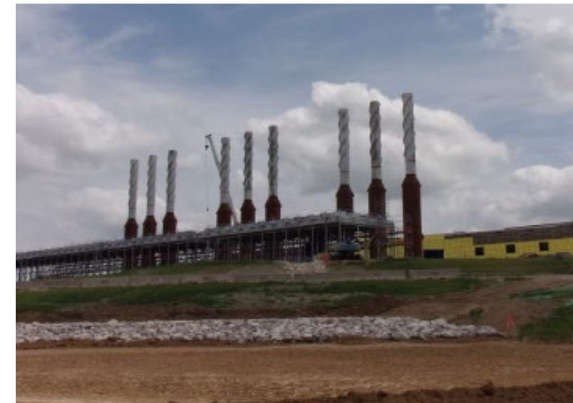
Facing Northeast – Radiators & Stacks
