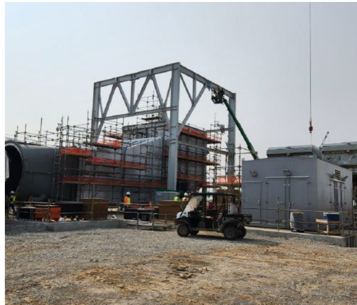
Facing Southeast – Unit #1 Stack
