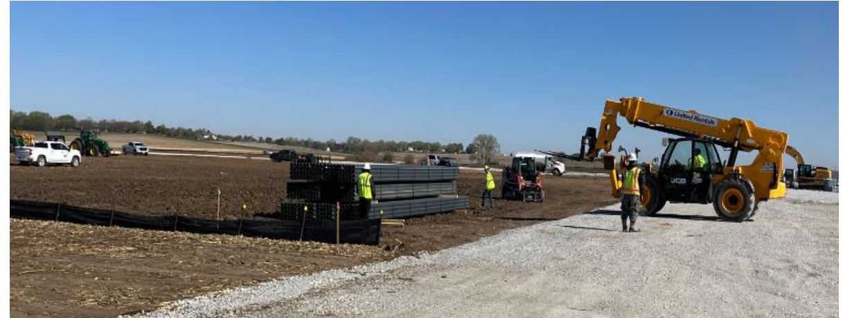
Platteview Solar – Material Staging
