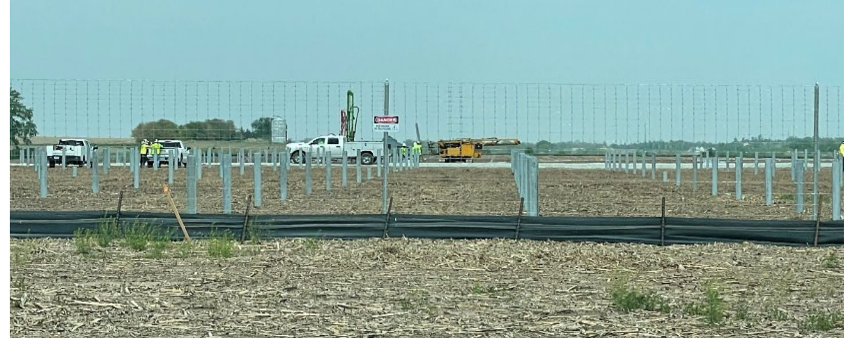
Platteview Solar – Piling Stands
