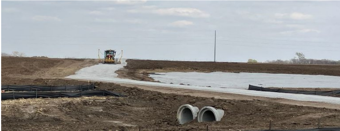
Platteview Solar – Access Road Preparations
