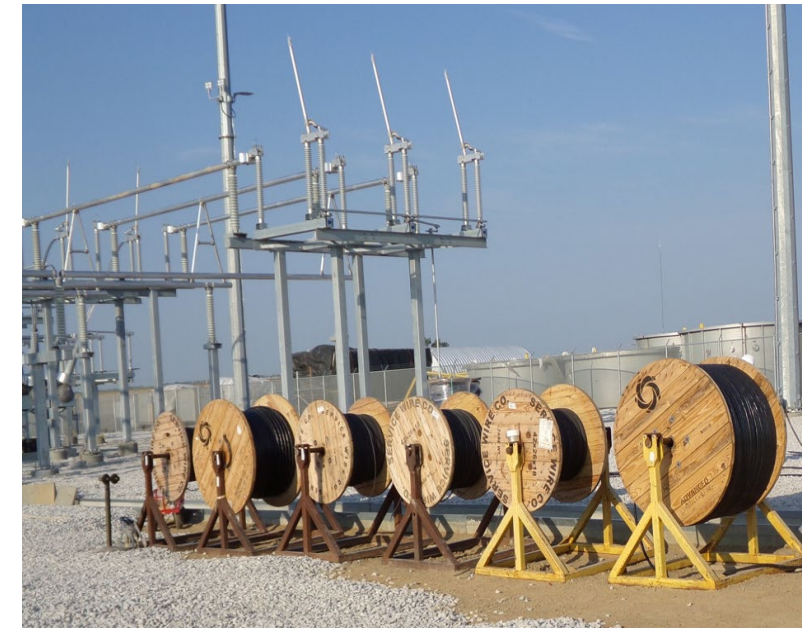
Substation – Cable Prep
