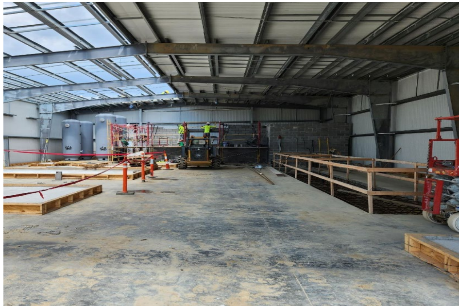
Water Treatment Building
