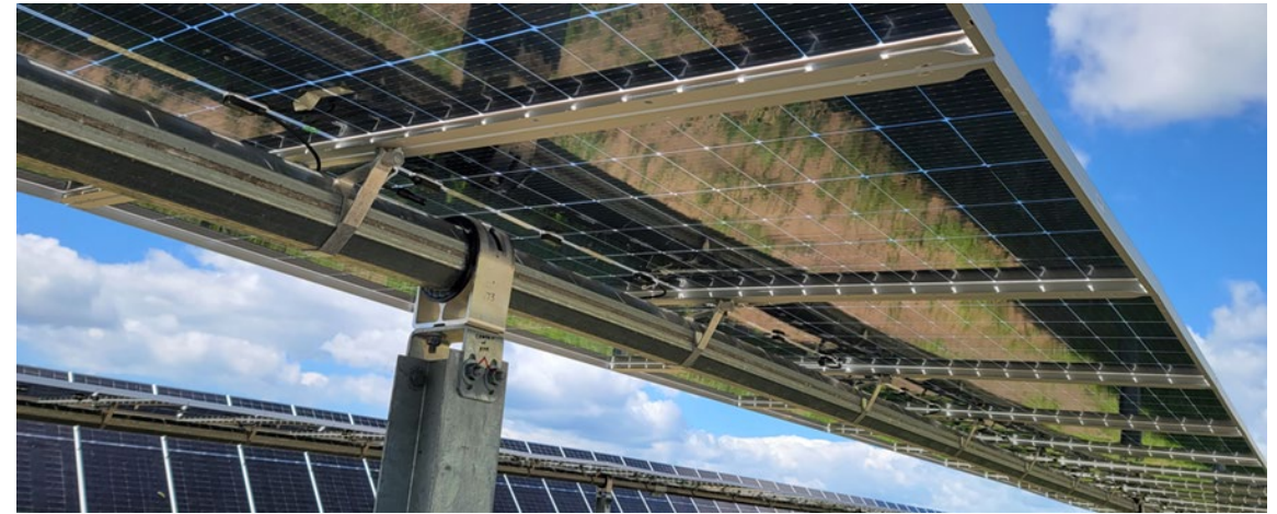
Platteview Solar – Racking & Module Installation
