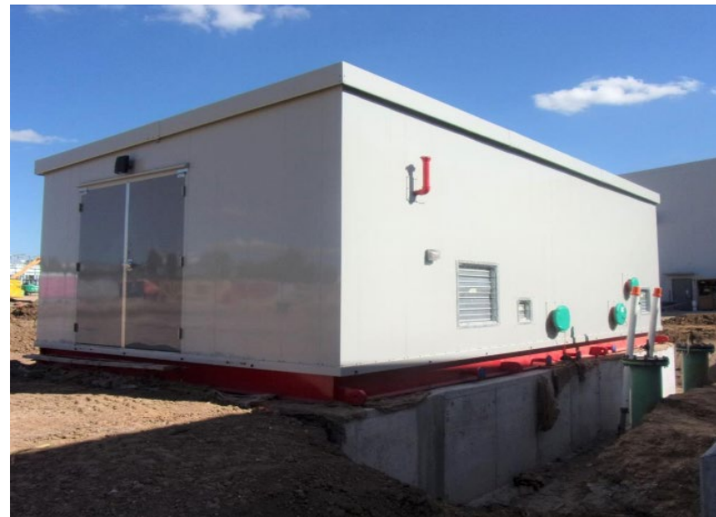
Facing Southeast - Fire Water Pump House
