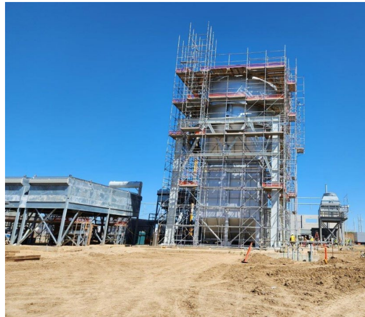
Facing North– Unit #1 Stack Erection
