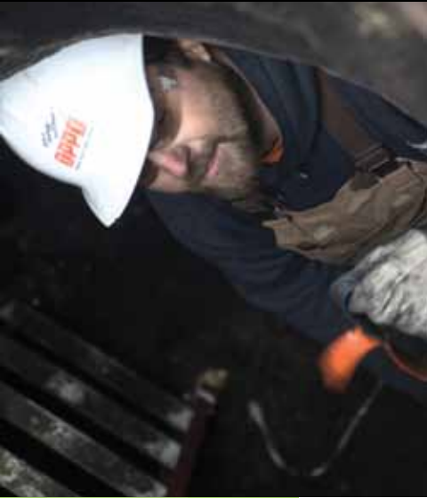
Cable splicer Scott Hadfield works in an underground vault in downtown Omaha. Earlier in 2012, seven other cable splicers (shown on the cover) spent two weeks in New York City to restore hurricane damage.
