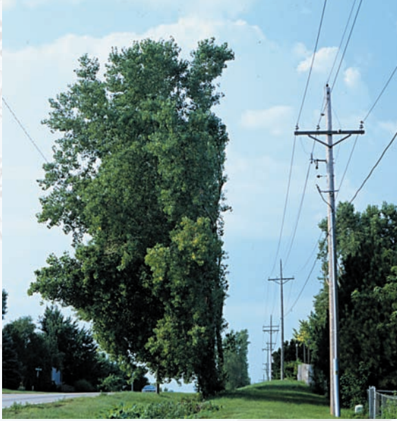
Side-trimming prunes back branches on the side of the tree.
