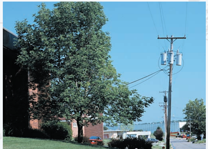
Notch-trimming prunes branches to create a “notch” in the upper tree crown so power lines can pass to the side and above the tree.
