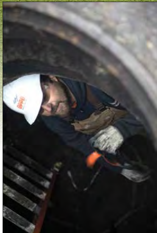
Scott Hadfield repaired an underground vault after a fire and explosion darkened a downtown Omaha business district.
