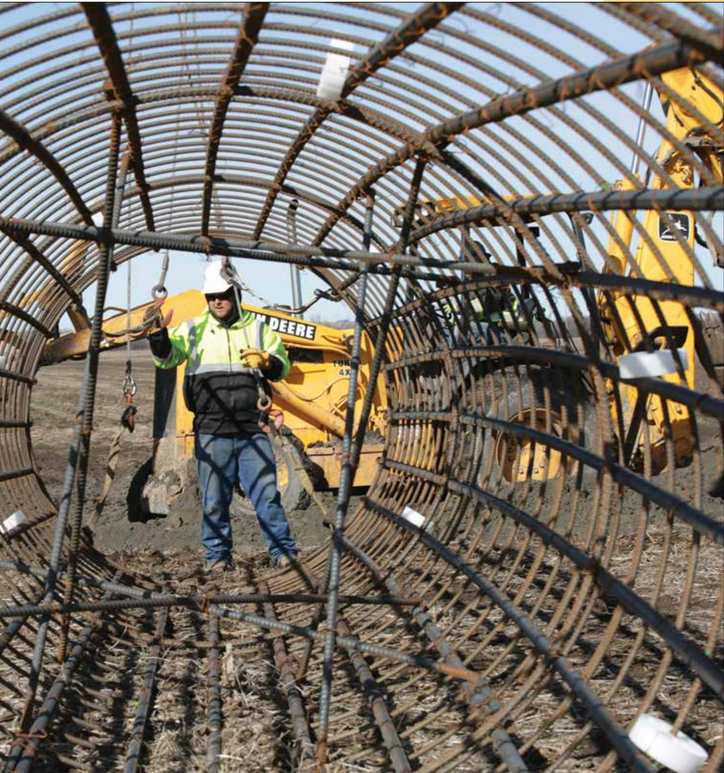
As part of being good stewards of customer-owner resources, OPPD executed a cost-effective plan for its 45-mile portion of the Midwest Transmission Project. The cost of OPPD's portion came in below the national average per mile of line. Shown above is rebar for one of 267 transmission tower footings. The Southwest Power Pool will reimburse approximately 95 percent of the cost over 30 years.
