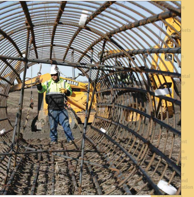
As part of being good stewards of customer-owner resources, OPPD executed a cost-effective plan for its 45-mile portion of the Midwest Transmission Project. The cost of OPPD's portion came in below the national average per mile of line. Shown above is rebar for one of 267 transmission tower footings. The Southwest Power Pool will reimburse approximately 95 percent of the cost over 30 years.
