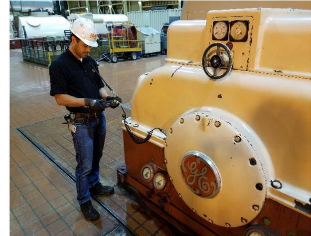
Engineer monitors vibrations on a generator exciter at North Omaha
