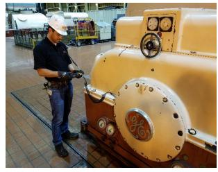
Engineer monitors vibrations on a generator exciter at North Omaha
