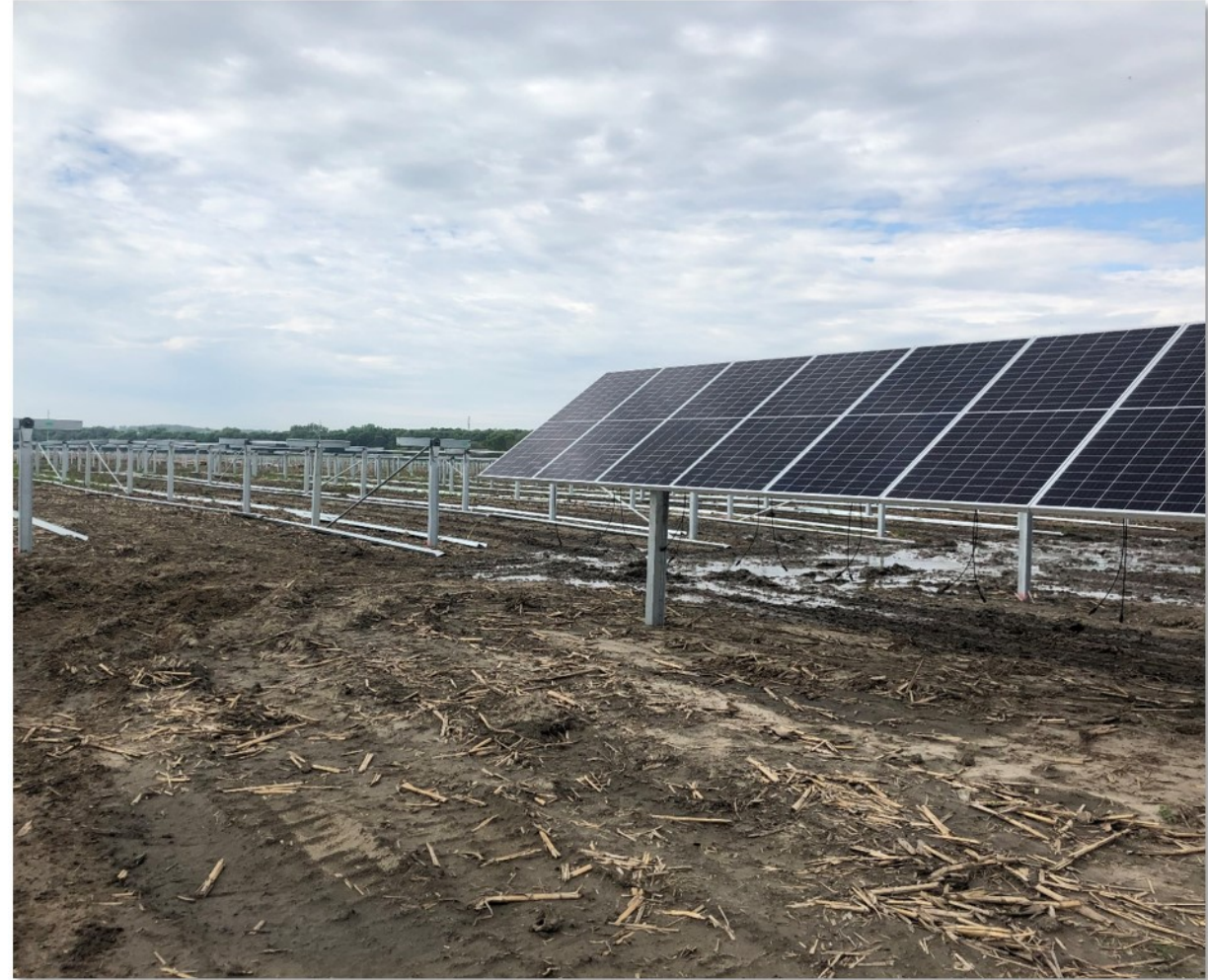
Photo shows solar facility construction at Fort Calhoun Community Solar
