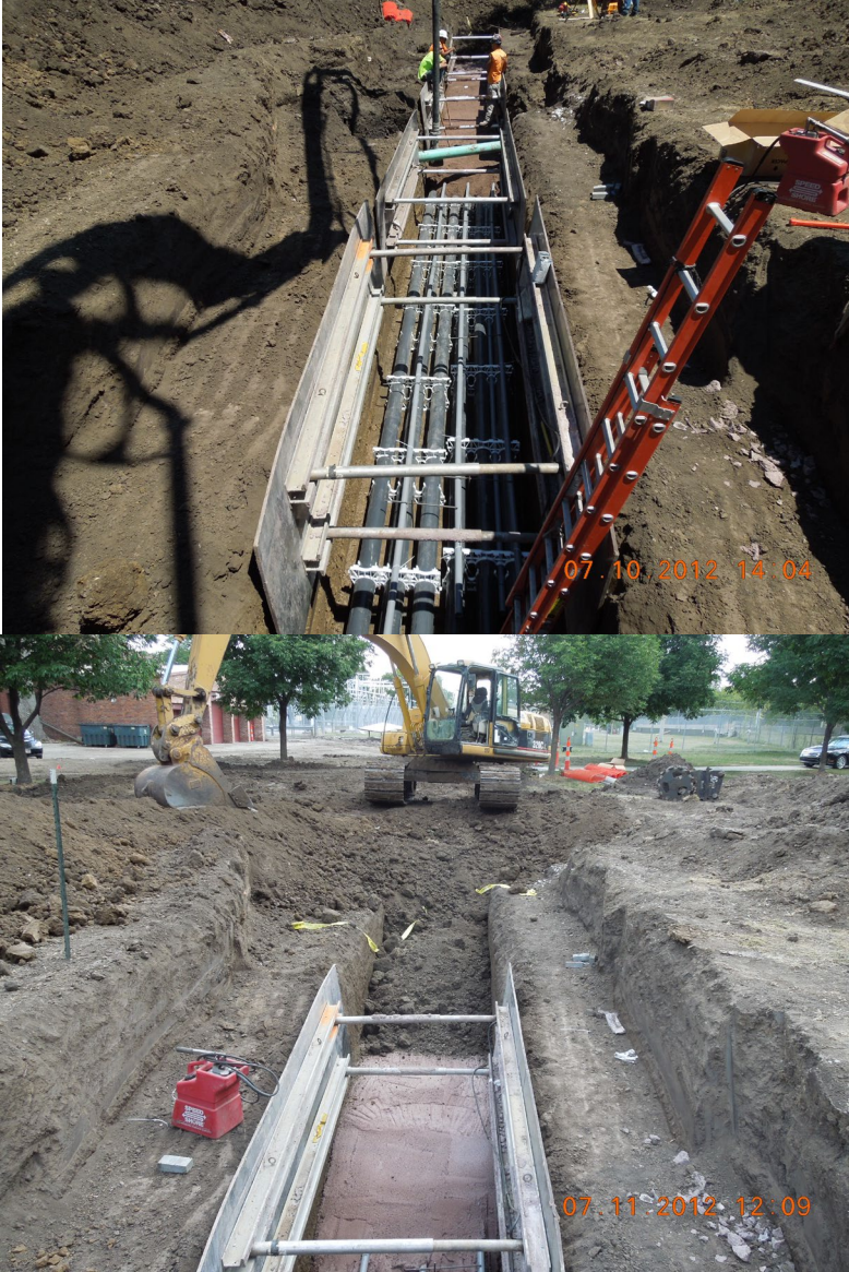
Ductbank Construction (EXAMPLE)
