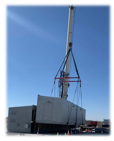
Control Building Enclosures house equipment to monitor, control, protect, operate, and maintain the energy delivery system.
