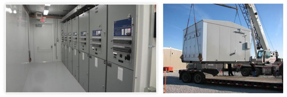
15kV metalclad switchgear cubicles house the 15kV circuit breakers and relay equipment to protect the distribution circuits and substation transformers. The enclosure keeps the switchgear out of the elements and provides area for electricians and relay techs to operate and maintain the switchgear, 15kV circuit breakers and relays.
