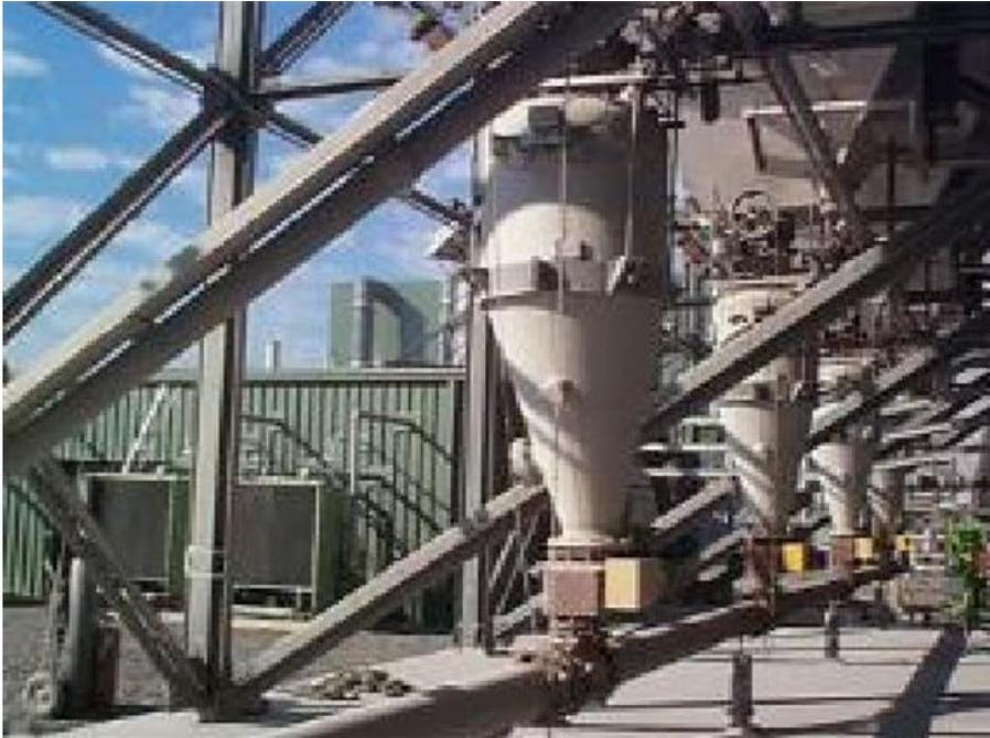
Example of new ash feeders and pneumatic transfer pipe
