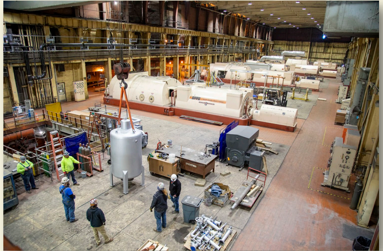
Work on a North Omaha Station auxiliary boiler in 2024
