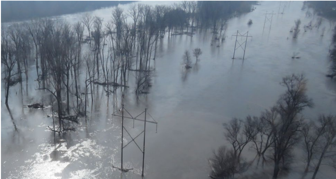
Figure 6-3 2019 Flood, Transmission Structures in water by the Elkhorn River, Nebraska
