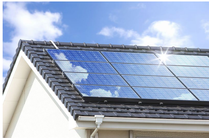
Figure 5-3 Customer-owner Distributed Generation. Solar Panels
