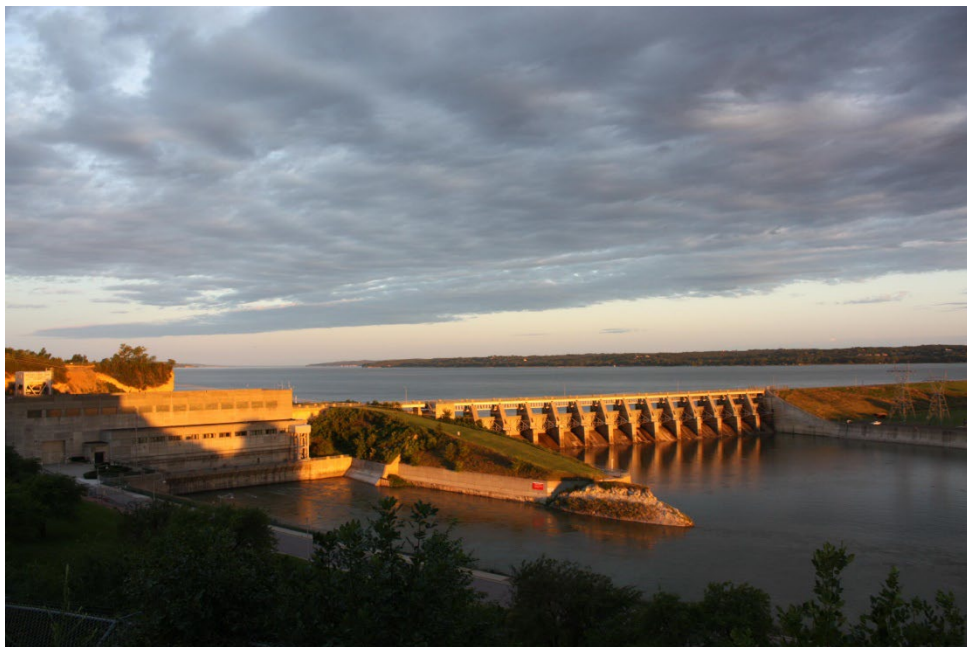
Figure 5-72 Gavins Point Dam, hydroelectric facility (Photo credit US Army Corps of Engineer)
