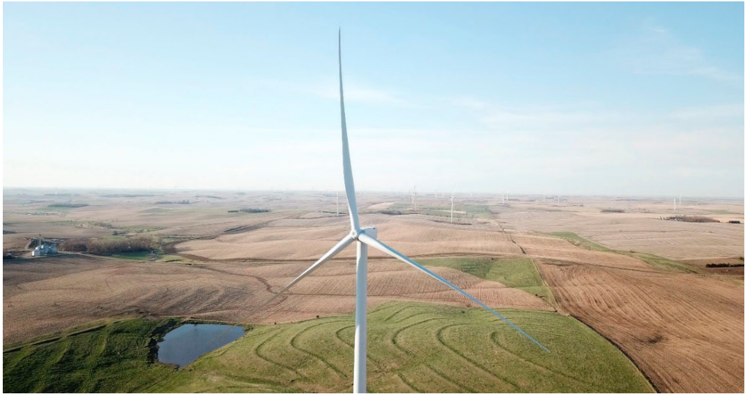
Figure 5-8 Sholes Wind Facility
