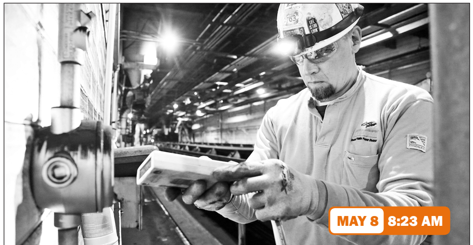
Wade Hatzenbuehler, combustion turbine technician, is among the many trades people, such as electricians, welders and steamfitters, who constantly monitor power equipment.
