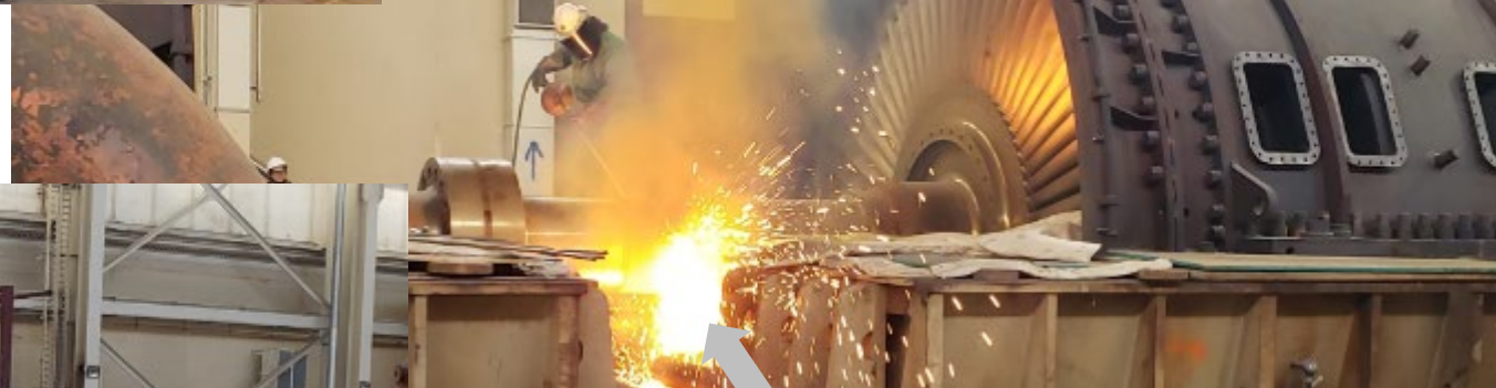
Cutting shaft between Sections 2 & 3
