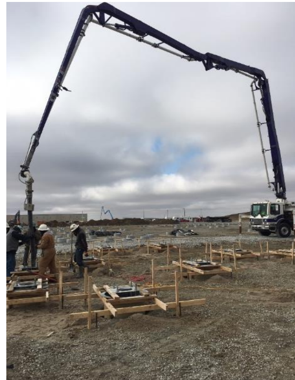
Pier Formwork
