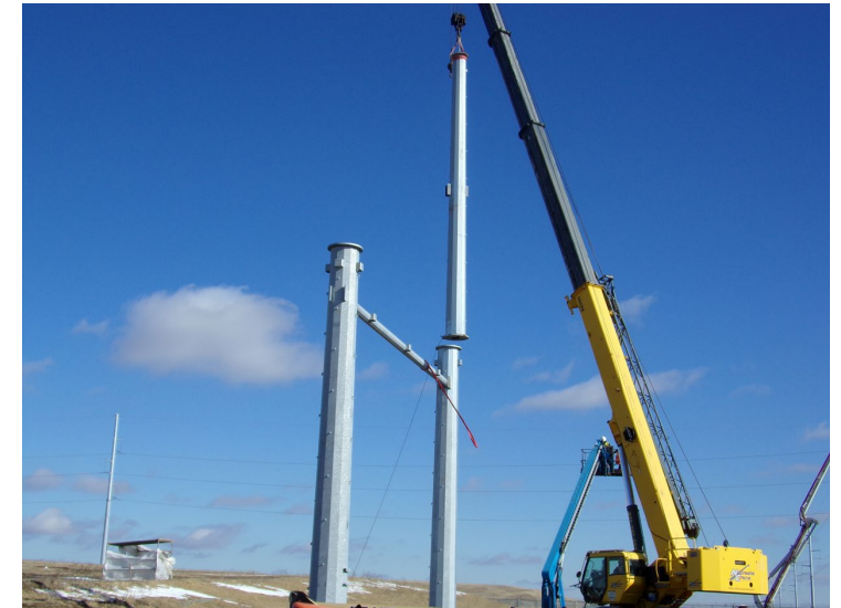
Substation H-Frame Erection
