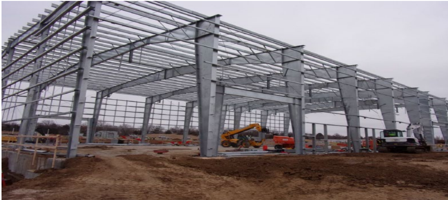
Facing Southwest – Engine Hall Enclosure Steel Erection
