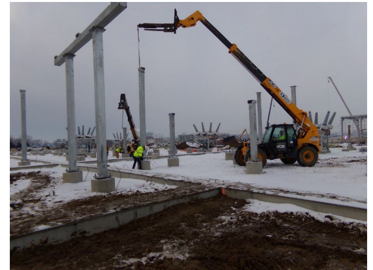
Substation Vertical Bus Support Erection
