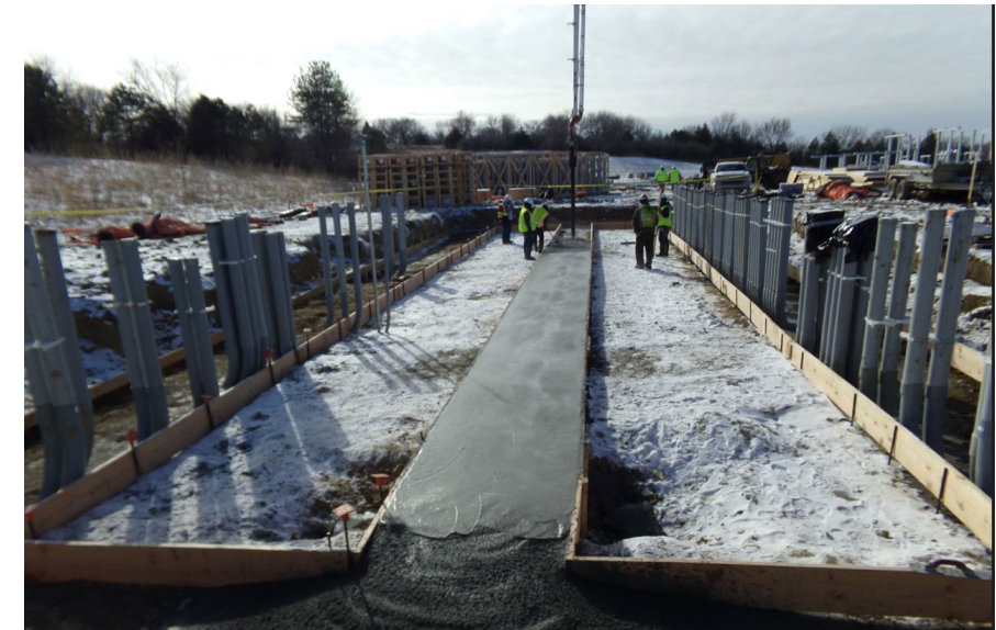
Substation Control House Foundation Prep Information as of February 3, 2023
