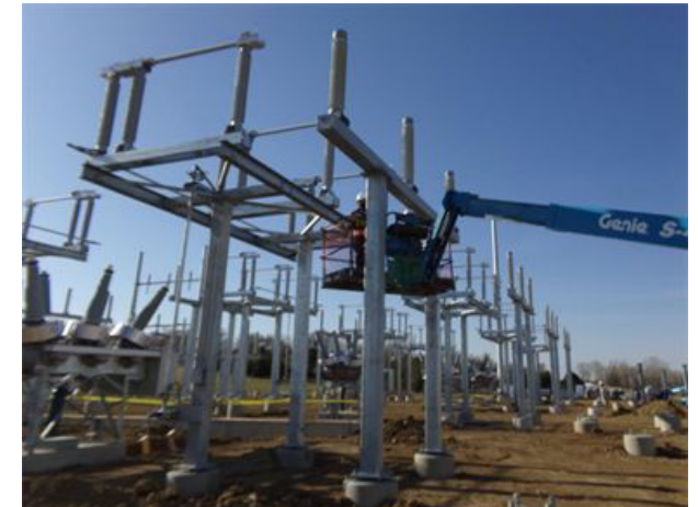
Substation – Horizontal Bus Installation
