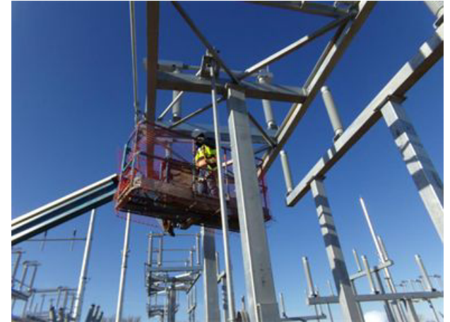
Substation – Horizontal Bus Installation
