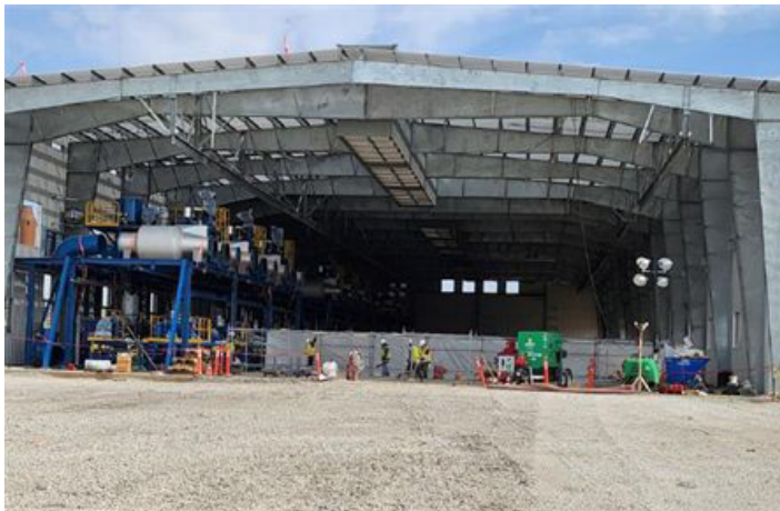
Facing North – Engine Hall Preparations & Installations
