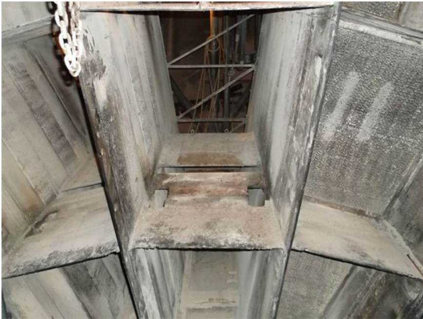
New baskets installed
