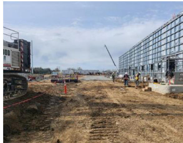
Facing South – On Site Heavy Haul Prep
