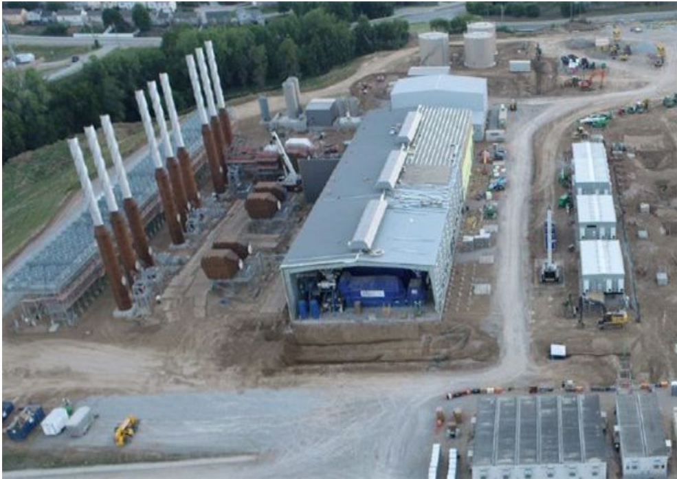
SBLs: Facing North, Aerial View
