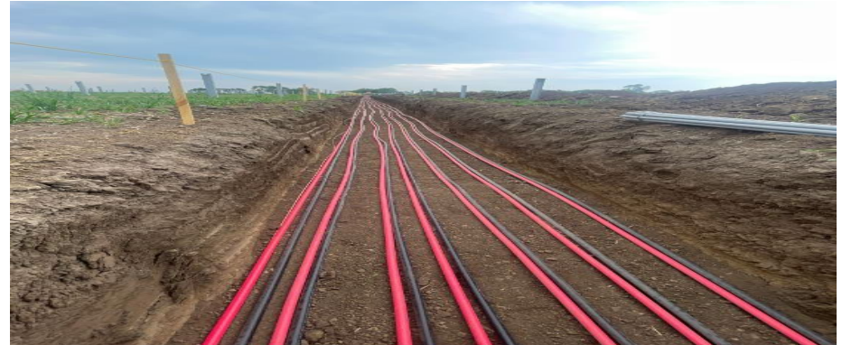
Platteview Solar – DC Trenching
