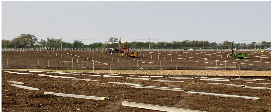
Platteview Solar – Pile Driving
