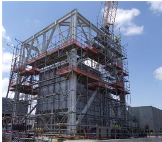
Facing Northwest – Unit #1 Stack Erection
