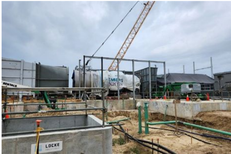
Facing Northwest – Unit #1 Turbine Enclosure
