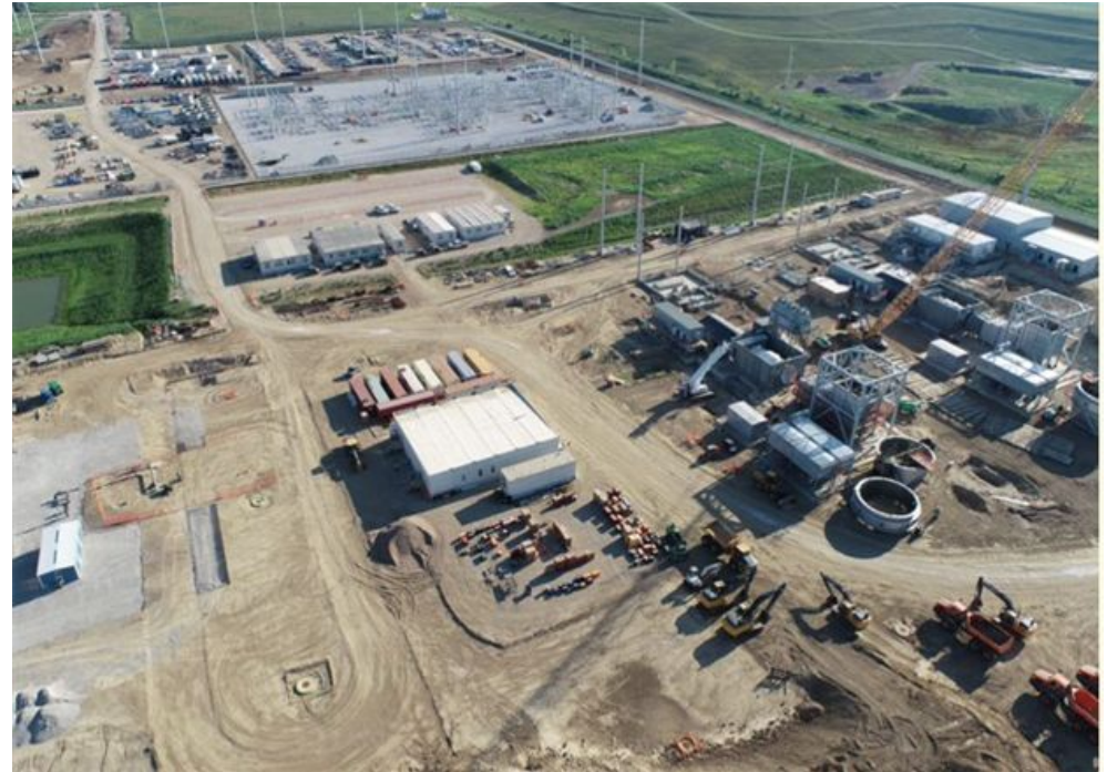
TCS: Facing Northeast, Aerial View
