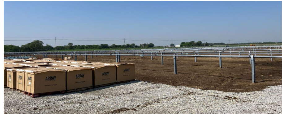
Platteview Solar – Racking Installation
