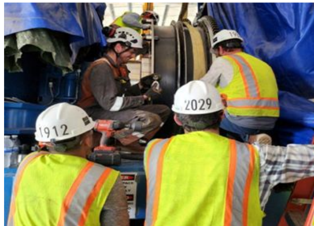
Engine/Generator Alignment/Coupling
