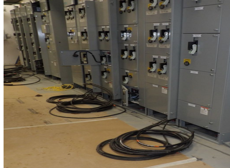
Electrical Equipment & Cable Installation
