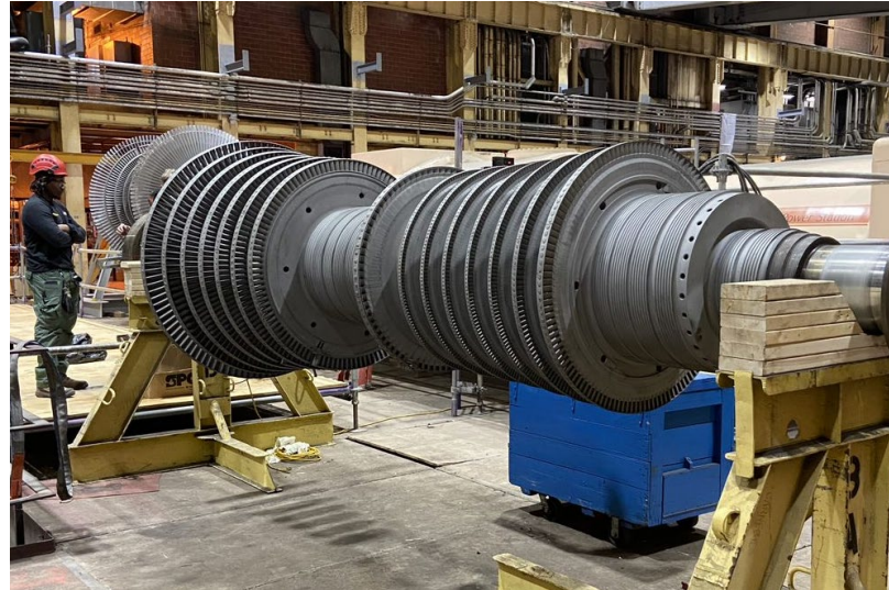
N04 Turbine Inspection
