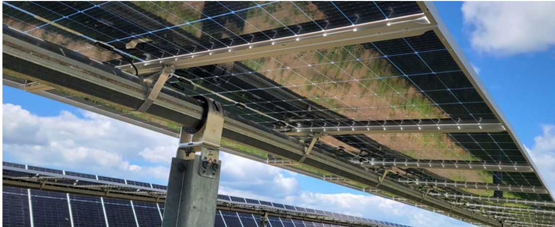
Platteview Solar – Racking & Module Installation
