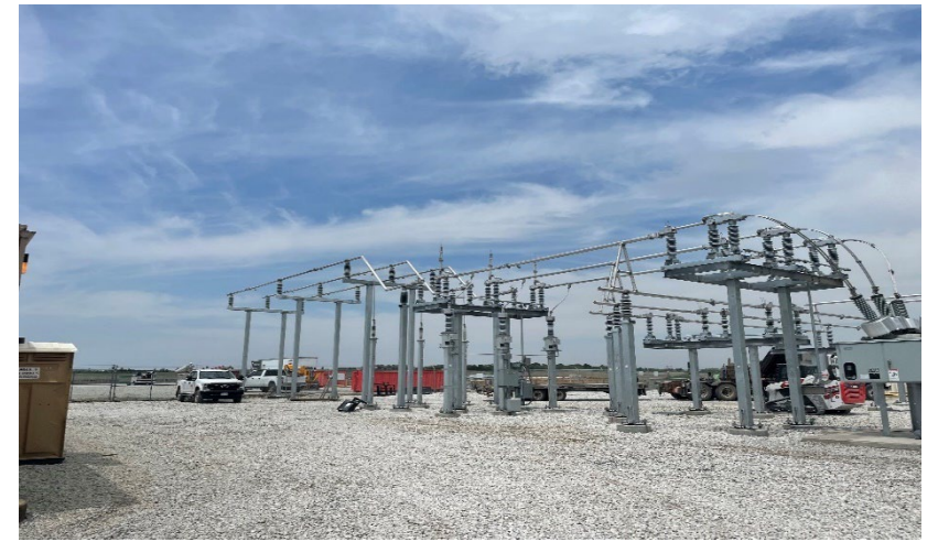
OPPD Substation – Bus Extension to AES Collector Substation
