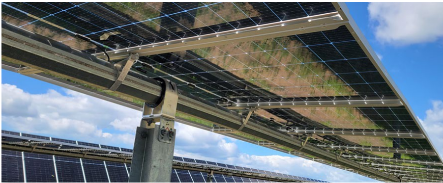
Platteview Solar – Racking & Module Installation
