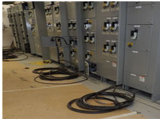
Electrical Equipment & Cable Installation
