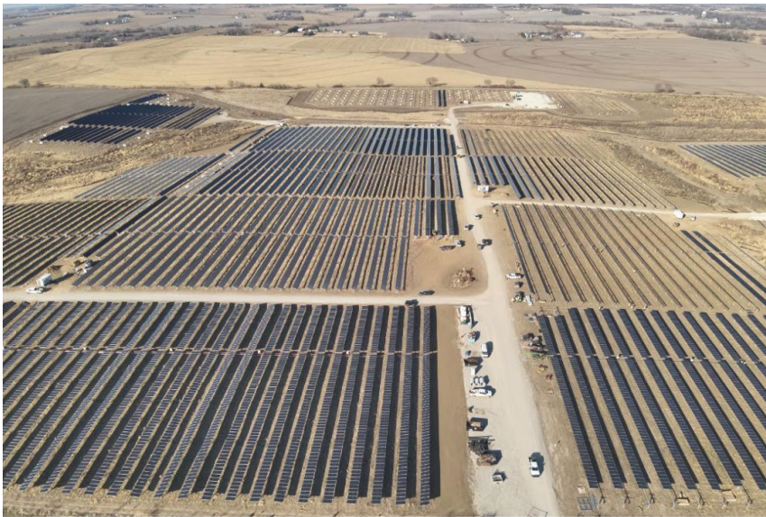
Platteview Solar – Aerial of North Parcel Dec 2023
