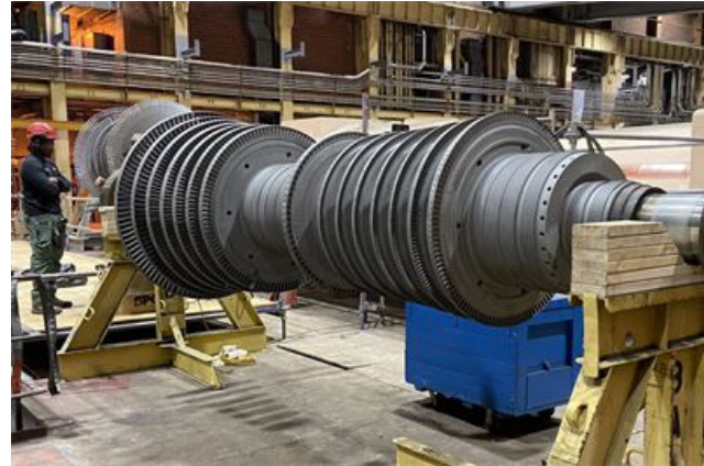
N04 Turbine Inspection
