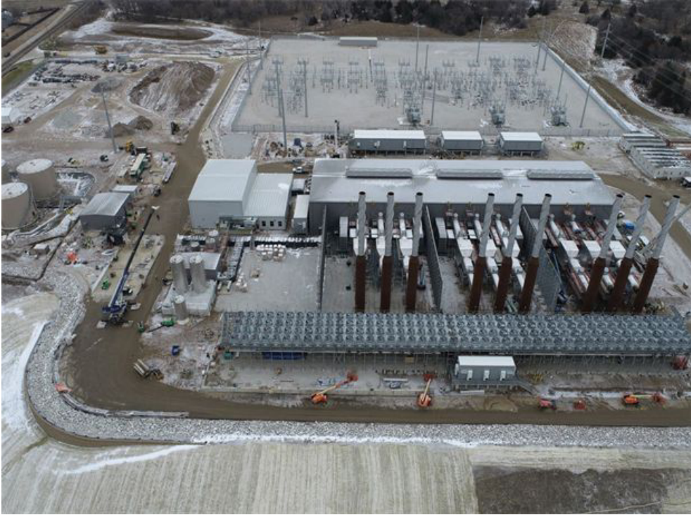
Facing East – Aerial SBLs, January 2024
